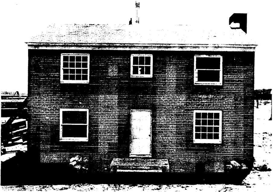
Figure 5.66. Unreinforced brick house before a nuclear explosion, Nevada Test Site.
