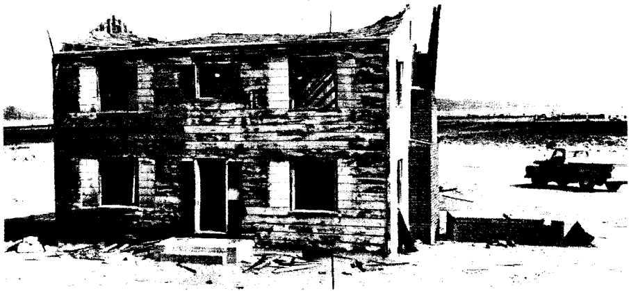
Figure 5.64. Strengthened wood-frame house after a nuclear explosion (4 psi peak overpressure).
