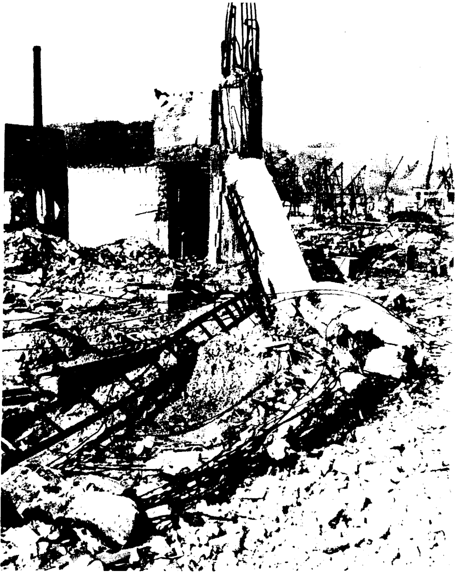
Figure 5.34b. A circular, 60 feet high, reinforced-concrete stack (0.34 mile from ground zero at Hiroshima). The failure caused by the blast wave occurred 15 feet above the base.
