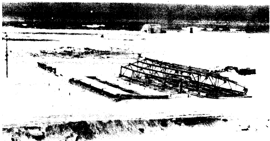
Figure 5.51b. Structure similar to Figure 5.48b after exposure to 5 psi peak overpressure and 0.5 psi dynamic pressure; positive phase duration several seconds.
